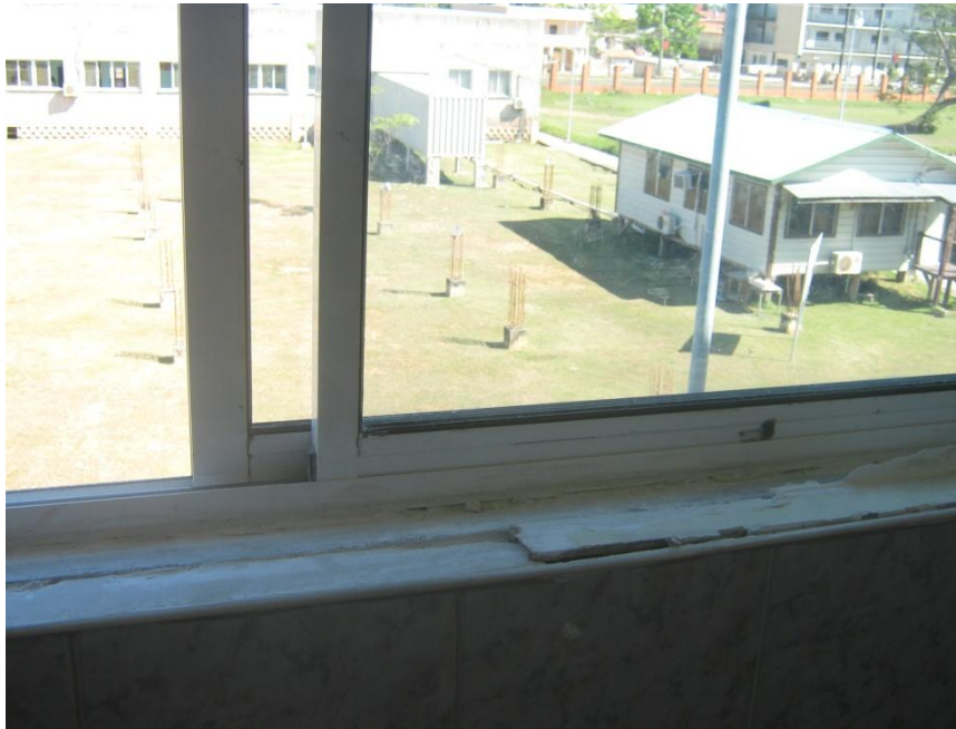
Deteriorating Window and Wall Works – #208
