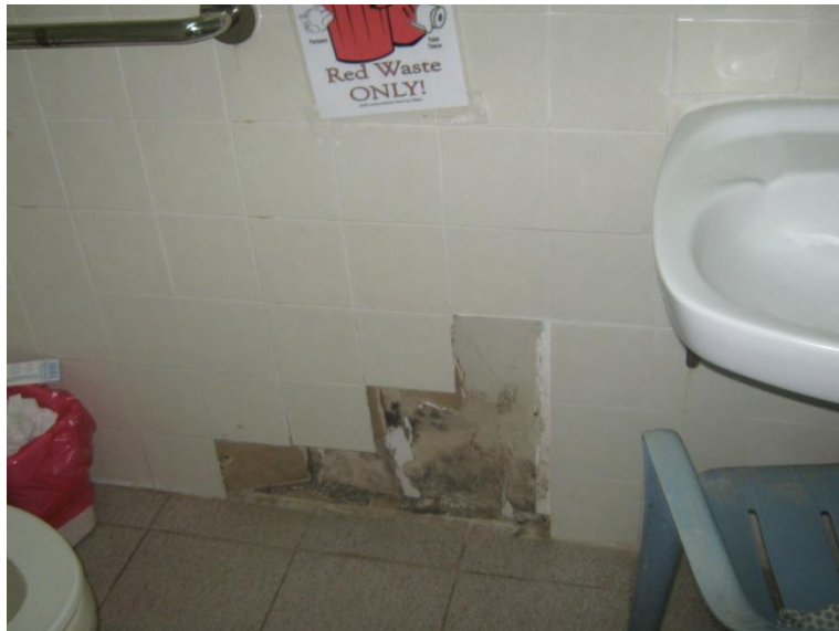
Example of Damaged tiles – #229
