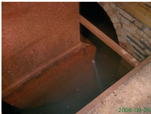
Water in base of furnace
