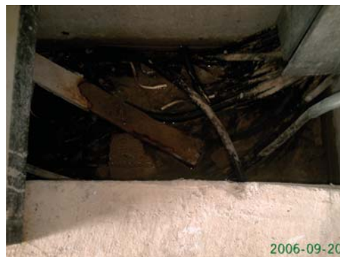
Electrical wires under water inside main control room
